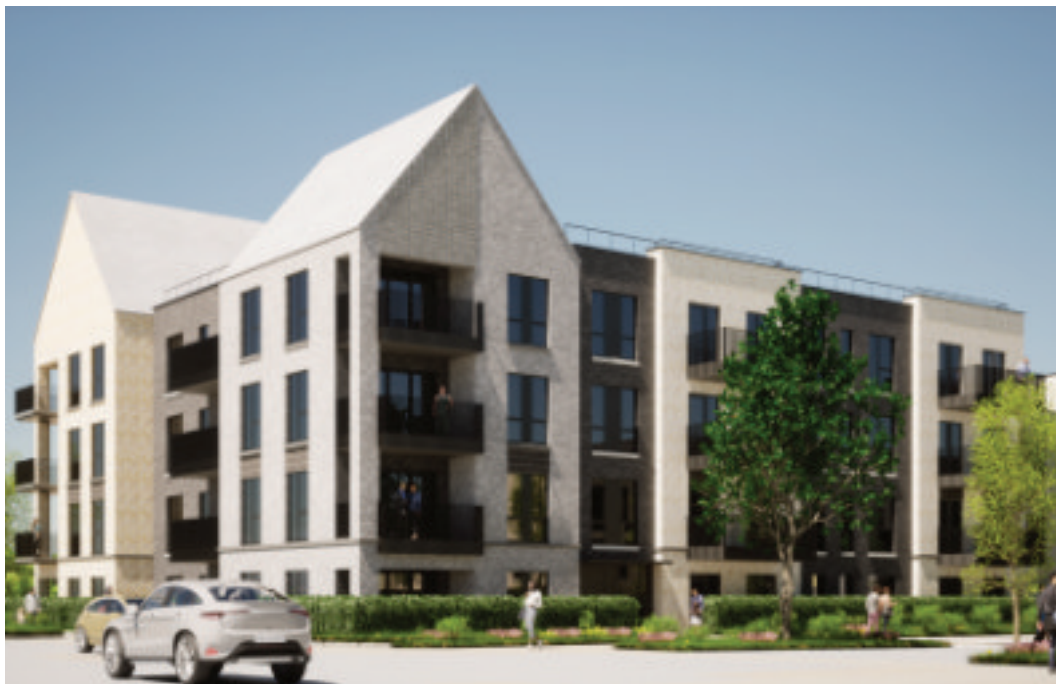
10.7 Apartment building developed from a simple block — cuts, shifts and varied roofs. / VISUALISATION
